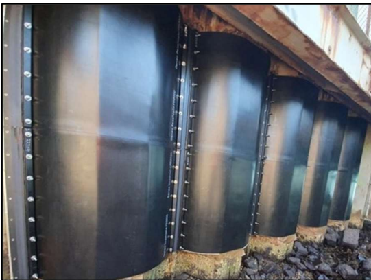
Figure 1. Completed system on a sheet pile wall.
