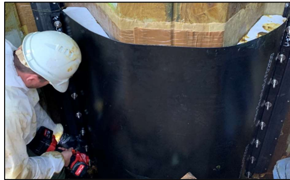
Figure 2. (1) Installation of the system; (2) note the petrolatum tape and rigid foam; (3) the worker is tensioning the outer covering.
